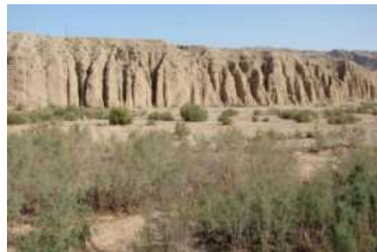
1b -Waterway Erosion
